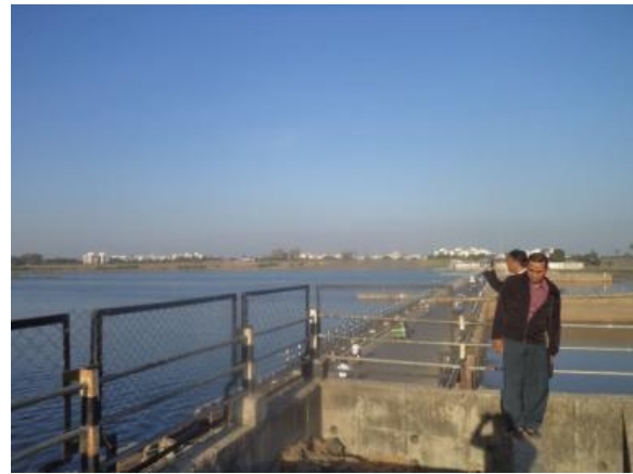
Delegation members during their visit to Weir-Cum-Causeway. Weir-Cum-Causeway, a drinking water supply source for Surat City.
