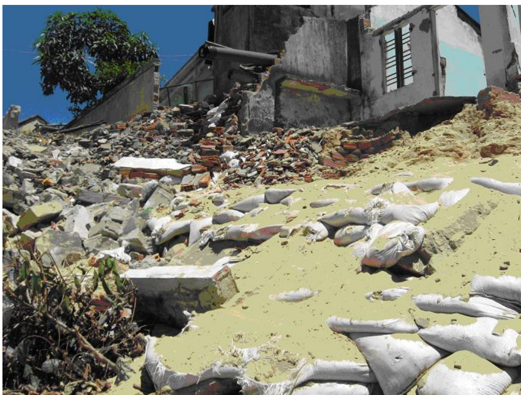
Where Mr. Sửu's house collapsed end of May 2009
